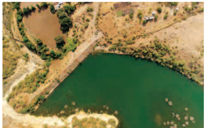
Water conservation through earthen dam construction
