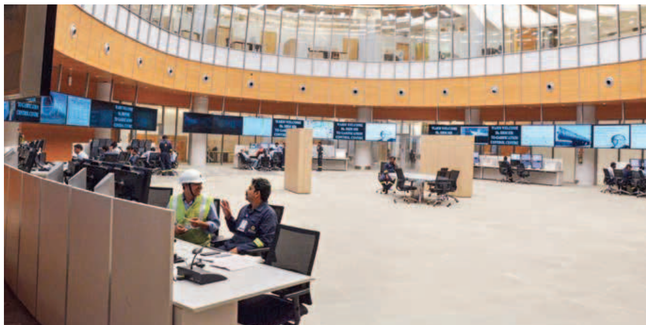
Cracker Control Centre at Jamnagar
