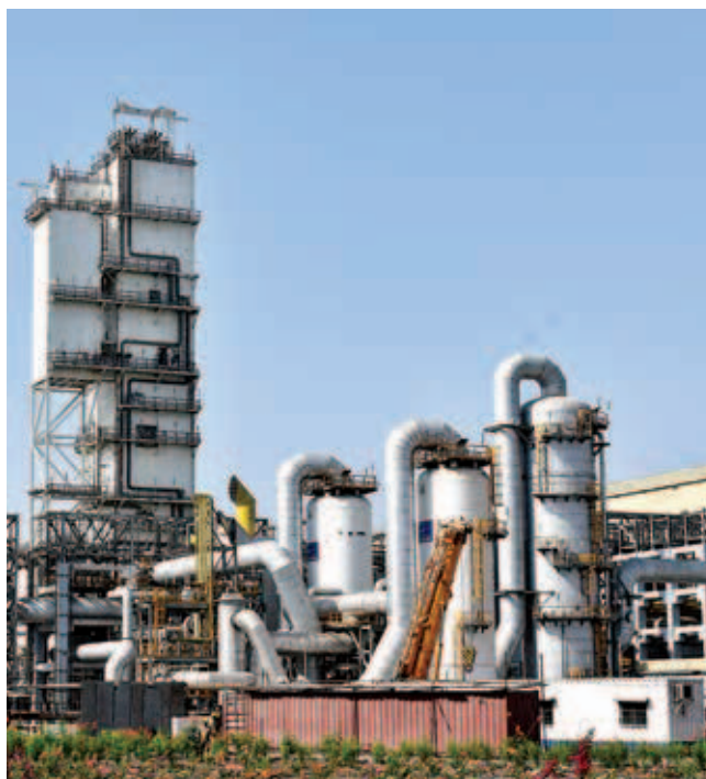
Gasification – Air Separation Unit
